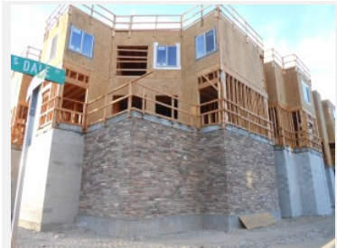
ZGA Architects is adding a rock veneer to La Pointe as a neighborhood enhancement. Photo by Teya Vitu
