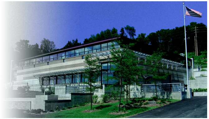
Exterior view of the completed heat exchange facility showing many of the architectural features.
