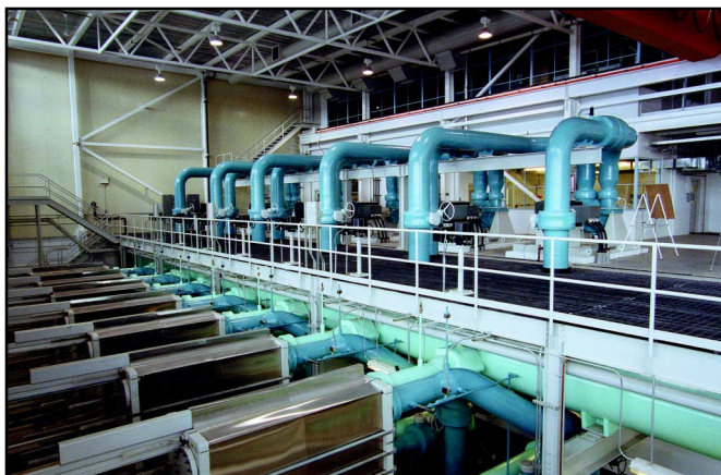
Interior view of the completed heat exchange facility.
